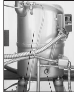
Compressor Crankcase heater
