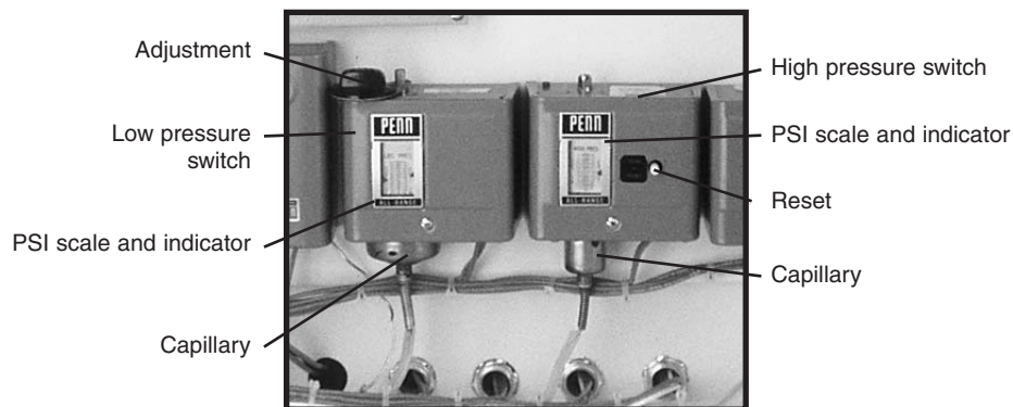
Low and high pressure safeties in separate housings
