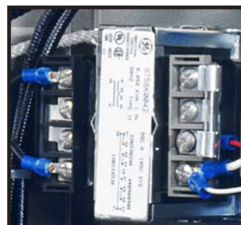
Control circuit transformer fuse Figure 2.5C
