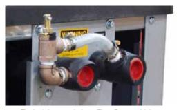
Typical Automatic Low Flow Bypass Valve
