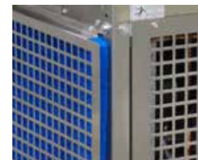
Typical Condenser Screen.
