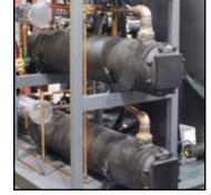
Water-cooled condenser. Configuration may be different on specific units
