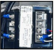
Control circuit transformer fuse Figure 2.5C
