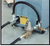
Typical pressure reducing valve Figure 2.2C installation (shown on S-925).
