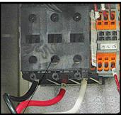
**DO NOT** reverse power leads Figure 3.2C at the unit's power entry
