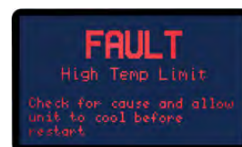
High Temp Limit Fault Screen.
