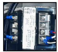
Typical control circuit transformer fuse
