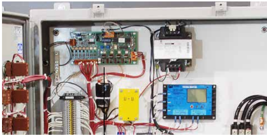
Typical Zone Board location inside electrical cabinet.
