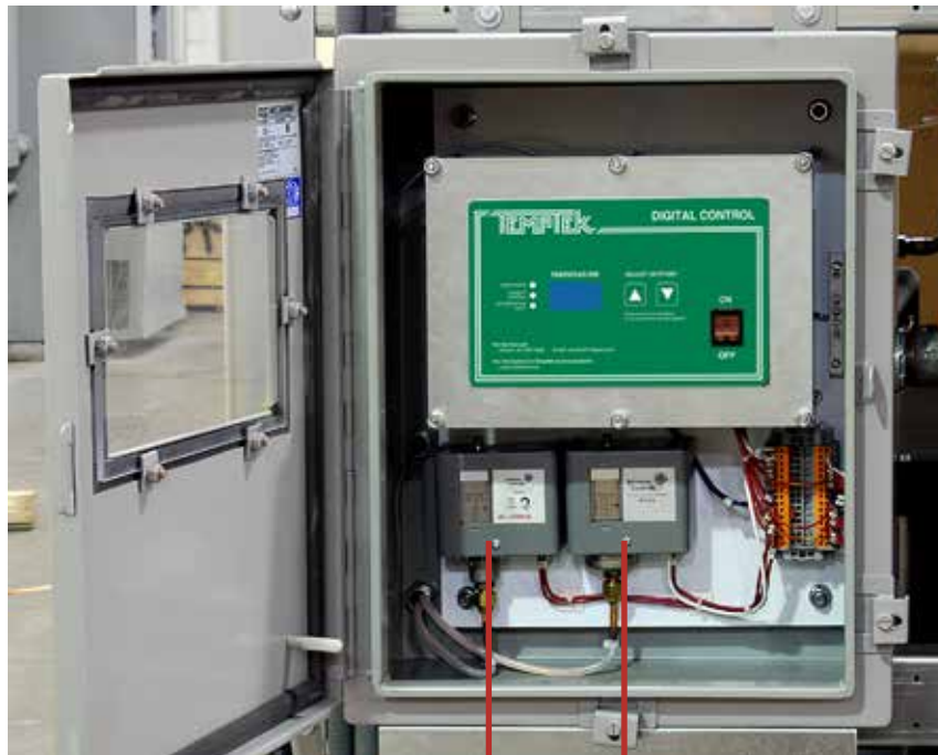
High Pressure Limit (Per refrigerant zone)
