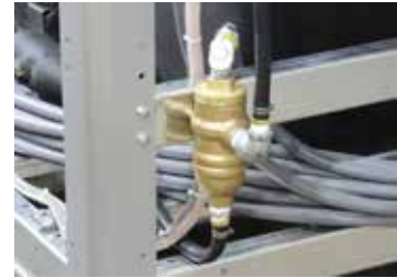
Typical water make-up level switch
